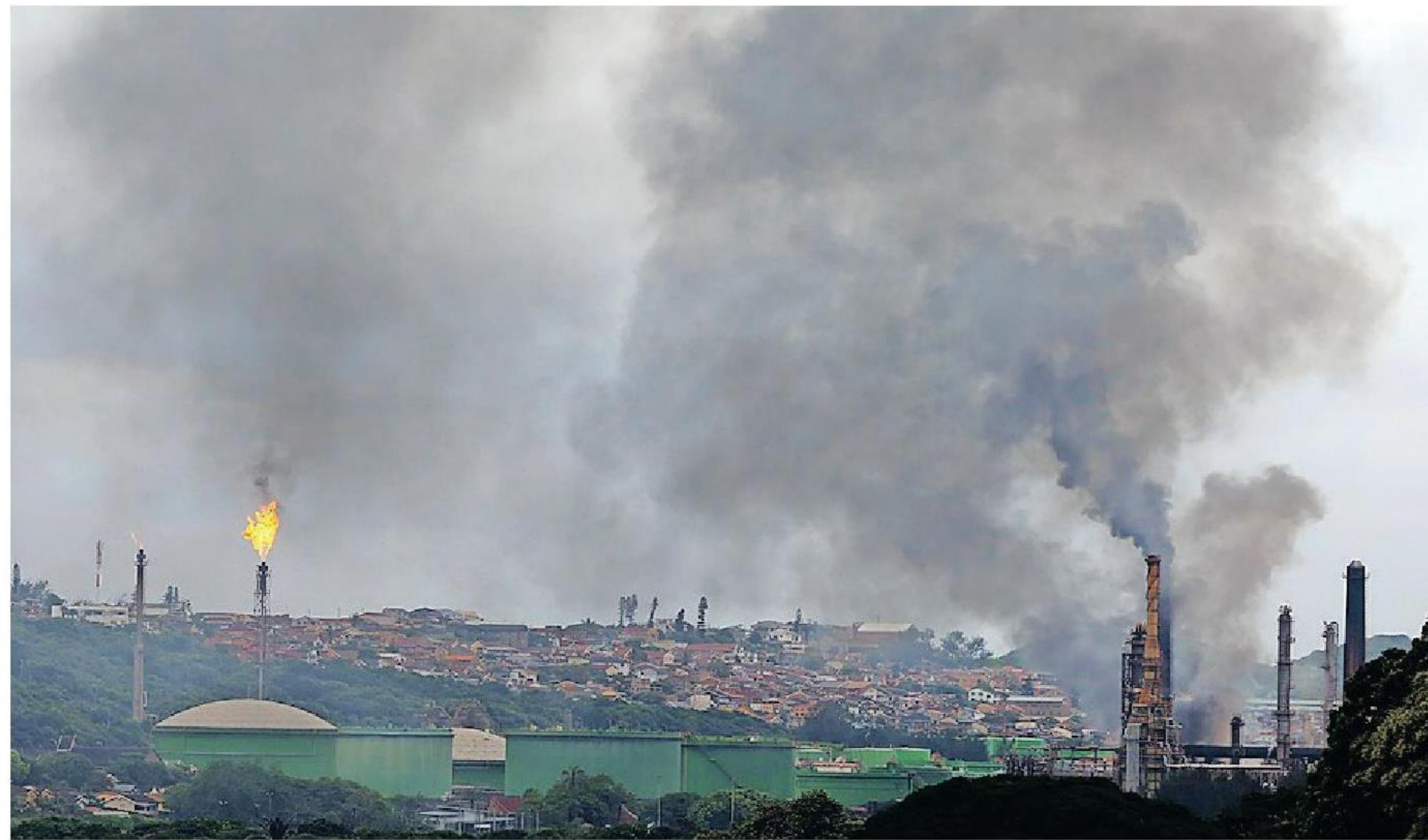
THE massive explosion at the Engen Oil Refinery south of Durban earlier this month was a culmination of a history of abuse of the environment and the people who live nearby, says the writer. | SHELLEY KJONSTAD | African News Agency (ANA)
